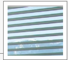
No visible vertical connections
